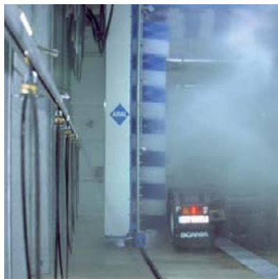
Hose-transportation in a truck washing facility
