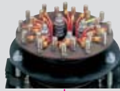
Wiring on clamping board
