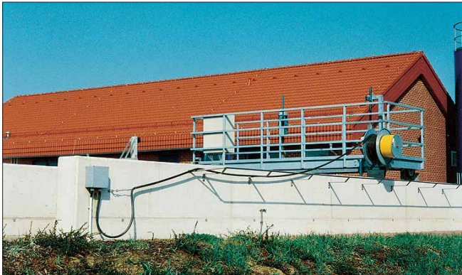
Main spring cable power feed for a skimmer in a water treatment facility.
