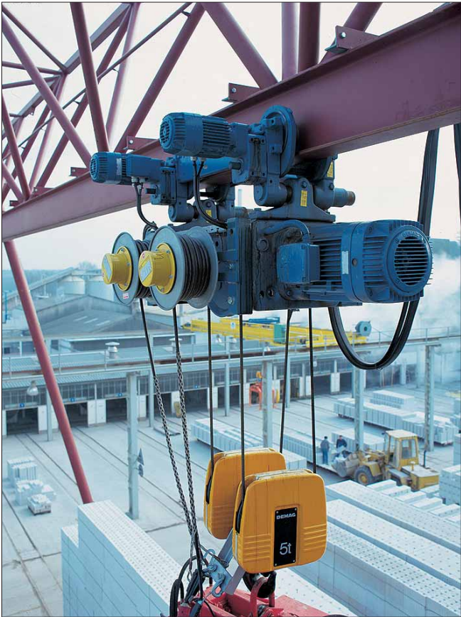
Portal crane with two spring cable reels for main and control current supply to the main grab.
