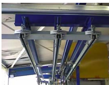
Underslung crane bridge
