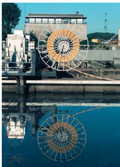
Cleaning up! The Sprinter motorized cable reel provides energy and data for a waste water treatment bridge.
